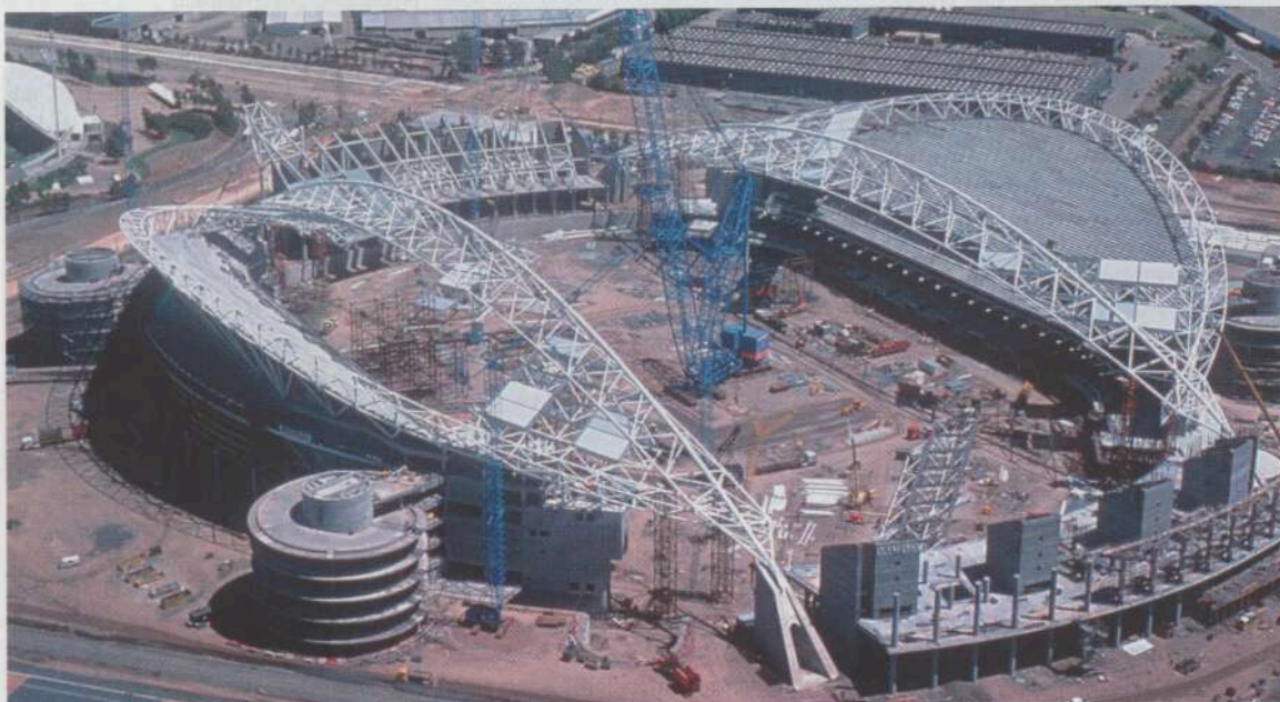
An aerial view of the Sydney 2000 main Olympic stadium during construction
