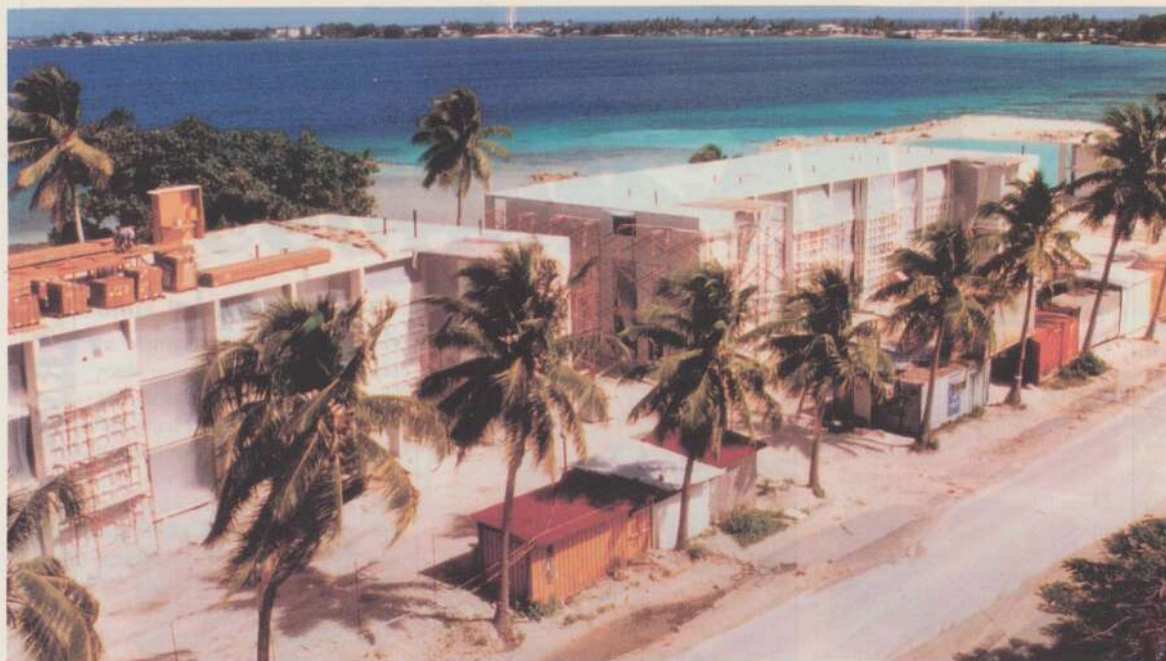
Construction of the hotel is providing temporary respite from the economic crisis
