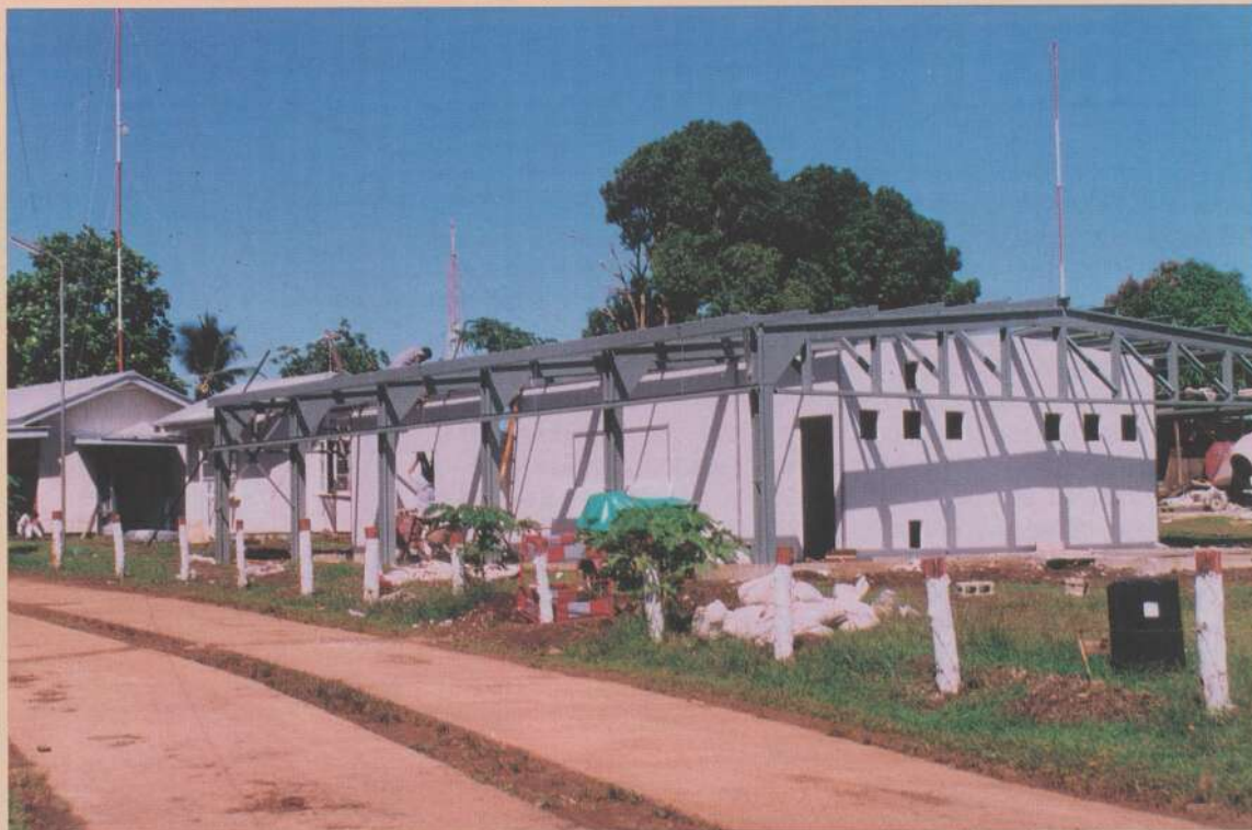
The earth station building at Ahau will provide automatic modern telecommunications services
