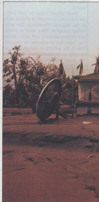
Telecommunications equipment destroyed at the Rabaul
