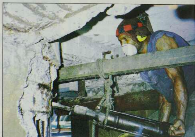
Foundations for the future: drilling the pile muffs at Lautoka wharf
