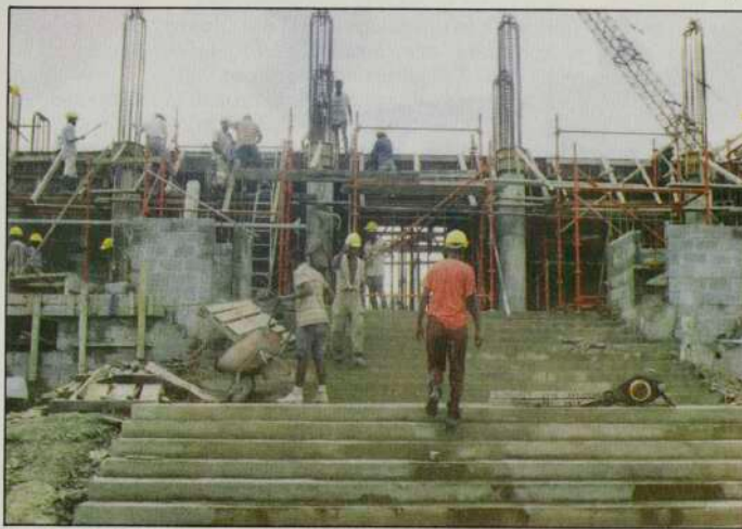
Going up: Fiji's new parliament house under construction in Suva
