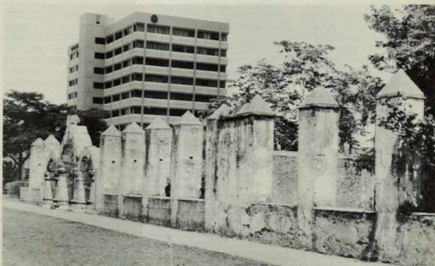
Past and present in Agaña, Guam: centuries-old walls from the Spanish colonial period are backed by the Chase office tower, symbol of U.S. financial might . . . Now for the future? — Paul Addison photo.
