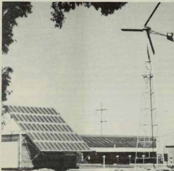
Experimental hybrid system for remote homesteads combining a photo-voltaic array consisting of 60 modules supplying 1.8 kW (electric, peak) and 5kW (electric) Dunlite windmill used in a project of the Solar Energy Research Institute of Western Australia (SERIWA). — Source, Solar Progress , July 1983.
