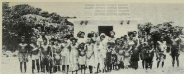
Fourteen Solarex photo-voltaic modules, supplying 500W (electric, peak) to a central system of a Solomon Islands village and its Community Centre — Courtesy Austin Dunsford, Solarex Pty. Ltd., Sydney.
