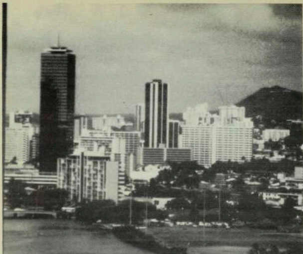
The high rise apartment and hotel buildings of Waikiki and its surrounding residential area jut high into an Hawaiian sky as blue as the brochures say it is.
