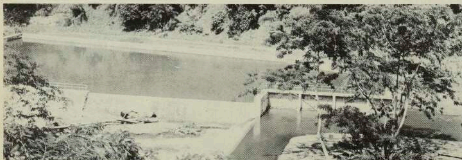
The headpond which supplies water for Samasoni hydro, 3¼ kilometres downstream.
