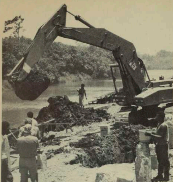
Workmen begin a feasibility survey to establish a pumping station which will increase the capacity of the Suva water supply. The project is part of Australia's aid commitment to Fiji.
