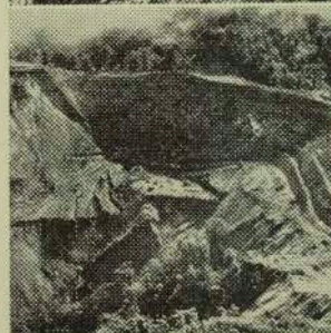
A section of highway under construction in the Crown Prince Ranges.
