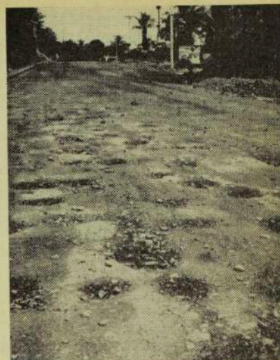
It's not necessary to drive along Queens Road to Nadi to experience bad roads. Mud and pot-holes pave the way in this street in Suva, capital of the soon-to-be dominion of Fiji.
