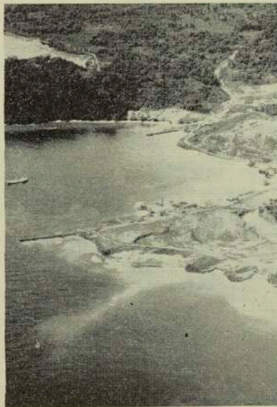
The new port takes shape at Anewa Bay. 40,000 tonners will come here. Area being levelled will be for bulk storage and wharf.
