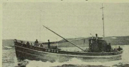
'Crystal Sea' Ring Netter built by Alexander Noble & Sons, Girvan, for Mr. J. Manson, Mallaig, propelled by Kelvin 240 shp TS6, Diesel.
