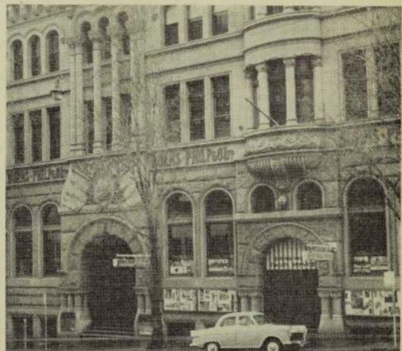
Seven Bridge Street, Sydney — BP's nerve centre. Cleaned on the outside, remodelled on the inside.
