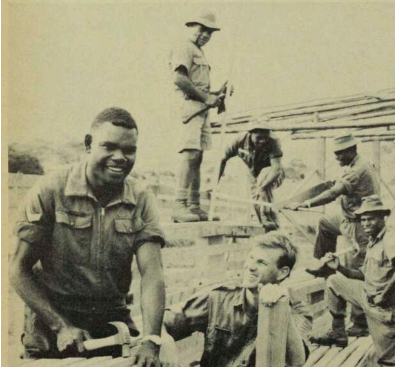
Cpl. Tovill, of Rabaul, and Sgt. K. Morcom, of Adelaide, supervise the building of a sports pavilion at Menyamya, P.N.G.
