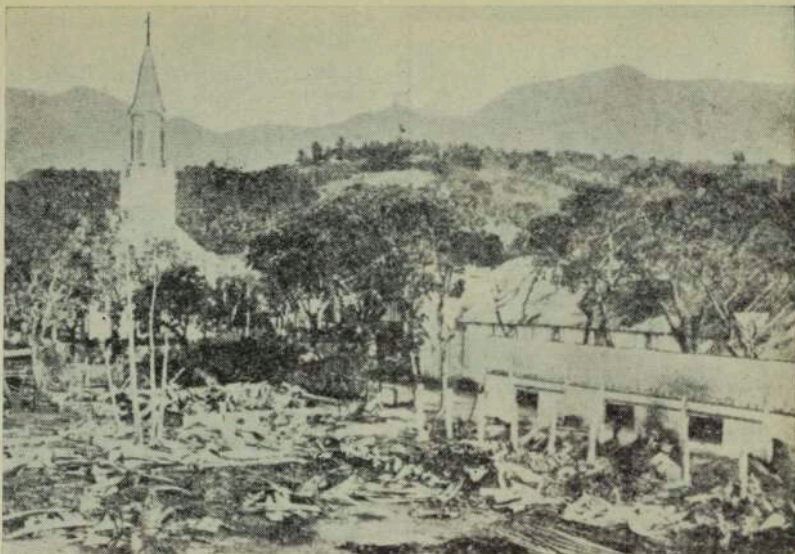
Damage caused by the shelling of Papeete by the "Scharnhorst" and "Gneisenau" in September, 1914.
