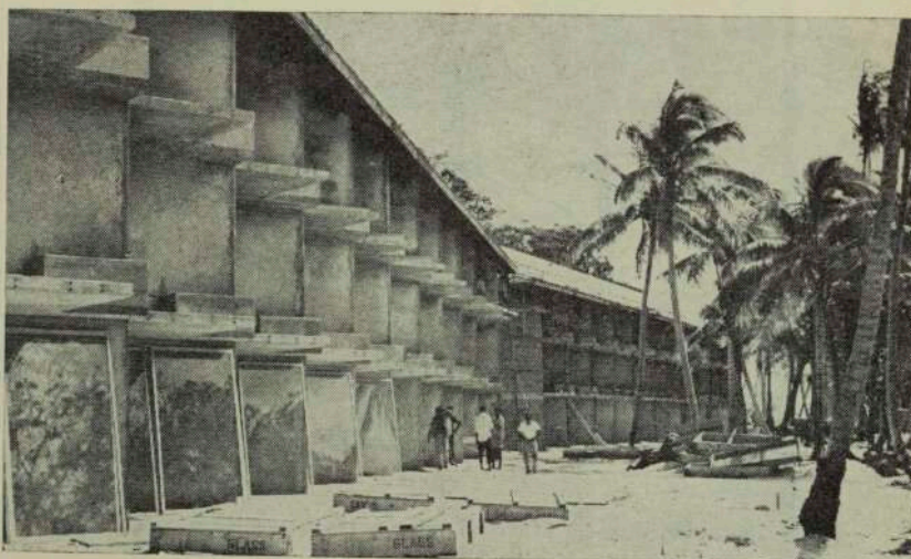
Is Fiji building too many hotels too quickly? There has been a big building boom in the last year or two. The Fijian, opened for business at the end of last year, is shown here when under construction; others continue to be built in other areas of Fiji.
