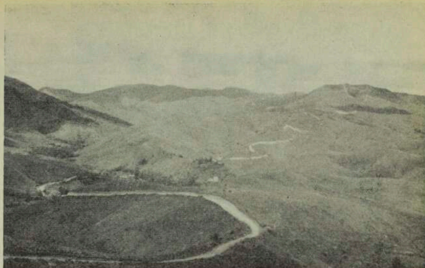
The road to the Highlands—the longest road in New Guinea. This typical winding stretch, cut into the hillside at many places, is between Kainantu and Goroka. The Highlands road is a growing tourist attraction, but travellers may still have their schedules upset by the weather.
