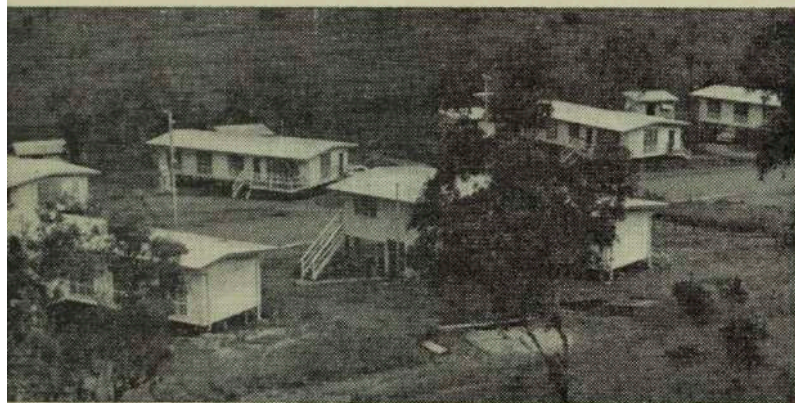
Papua-New Guinea probably makes more use of the traditional European house—built at great expense—than any other territory. These are at Boroko, a Port Moresby suburb. Experiments are now going on in P-NG into low-cost housing.
