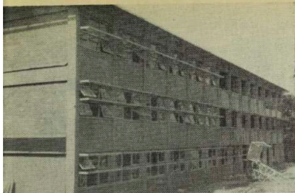
FIRST OF ITS KIND: This three-storey cement brick building stands out like a monument among all the fibro, tin and timber buildings at Konedobu, Port Moresby, the P-NG administration centre. When completed, it will be the first fully air-conditioned building at Konedobu.—Photo: Papuan Prints.
