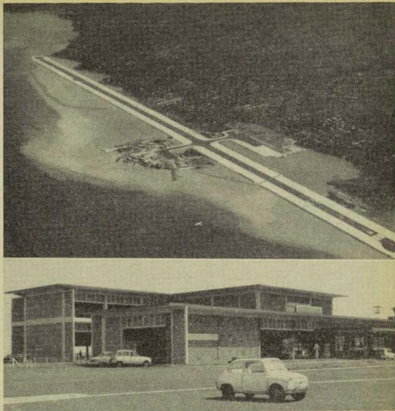
For Rarotonga to get into the international aviation picture, it would have to have a sealed airstrip like the one at Faaa, Tahiti (top), which was opened in 1961. The Faaa strip, 10,000 ft. long, was built by reclaiming the coral reef. It is only five miles from Papeete (on the bay at the top of the picture). Below is the newly-opened terminal building at Faaa. It replaced a temporary structure which had been in use since the airstrip was opened.—Photos: Courtesy of Qantas.
