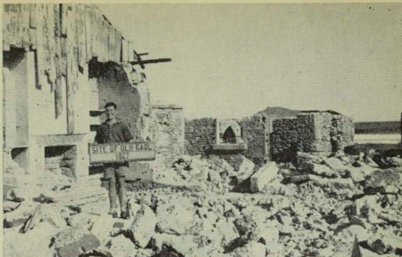
No one seems to be quite sure whether this old building, demolished last year, really was a gaol in Norfolk's convict days. What is left of the building is on the waterfront near Kingston Pier.—Photo: Ken Mullen.
