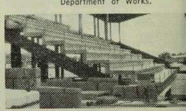
Monier pre-cast grandstand at Boroko Oval. Builder: John Stubbs.
