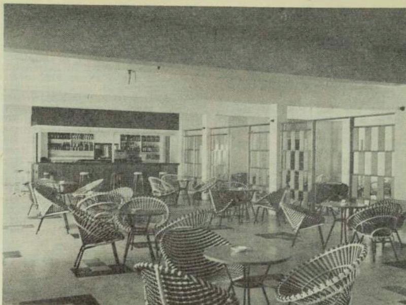
NEW HOTEL. This is the lounge of Cathay's new South Pacific Hotel, which opened for business at Lautoka, Fiji, in December. It has 25 bedrooms, including two suites, all with their own bathrooms and all air-conditioned. Photo: Stinsons
