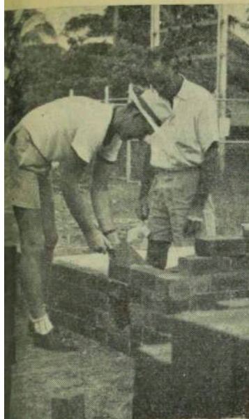
NG, building contractor and brick works, Charles Hyland (right) supervises a bit construction work on Lae's first brick building.
