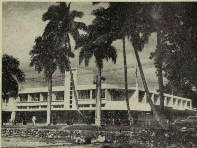
The new, luxurious Club Hotel, containing 18 air-conditioned rooms, at the corner of Victoria Parade and Gordon Street, Suva, Fiji, which was officially opened on December 1. This photograph was taken from the water-front. The western section (left of picture) looks out over Victoria Parade, onto the harbour; the main entrance is in the right-hand section, facing Gordon Street.
