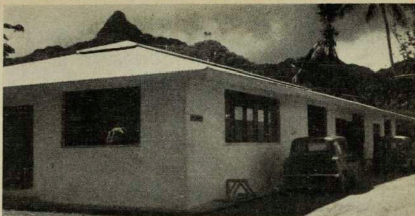
This is a handsome example of coral-lime construction which is becoming a popular building method in the South Pacific. The building is for the Social Development staff of the Cook Islands' Administration, and has recently been finished at Rarotonga. Photograph below shows experimental bricks manufactured by the Department of Works in Lae, N.G.
