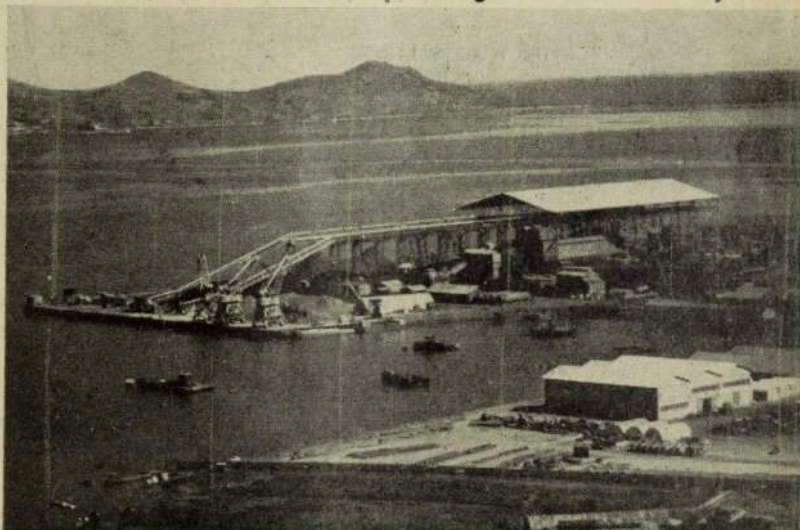
The new unloading installations at the Nickel Co. in Noumea, New Caledonia. The ore is removed from the ships on endless belts and is carried into the hanger where it is prepared for smelting. Ile Nou, once a notorious convict settlement, is shown in background.
