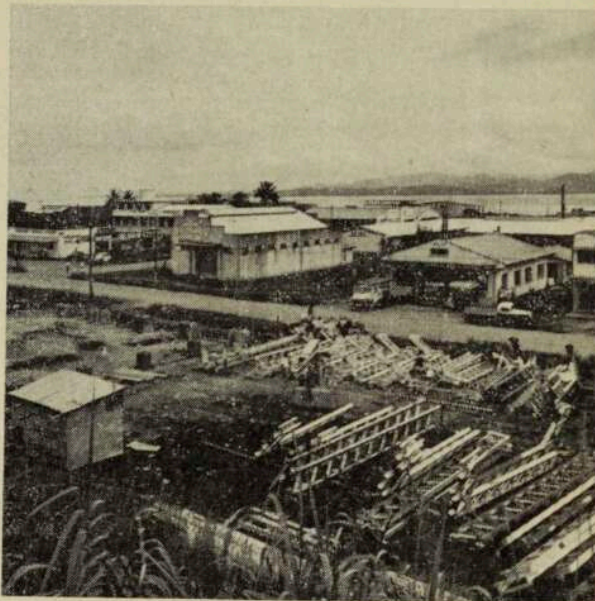
In foreground—the beginnings of the new Suva brewery at Walu Bay. Photo: Stinsons.
