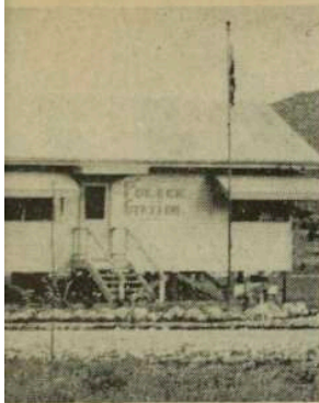
Completed Police Station at Bulolo, Photo: N. Brady.
