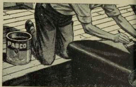
Fix and dress Malthoid with Pabco Cement and coating. You'll get dependable protection rugged efficiency against storms and sweltering heat.
