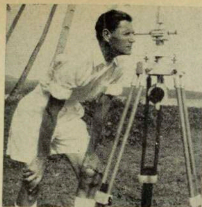
Mr. A. L. Burrows, director of the Apia observatory, peers into a theodolite as he tracks a balloon to determine upper air movements—one of the operations in present Pacific hurricane forecasting techniques. Expensive radar stations have replaced some theodolites—but inexpensive microseismic stations may supersede radar, as this article explains.
