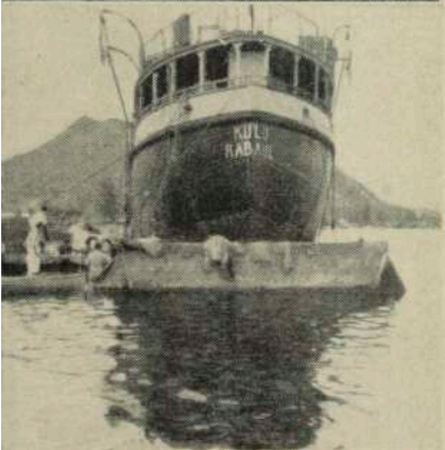
Top: Mr. Mike Morgan, inside the cofferdam, at work on the "A" brackets. Lower: The Kulu with her stern supported by the cofferdam.
