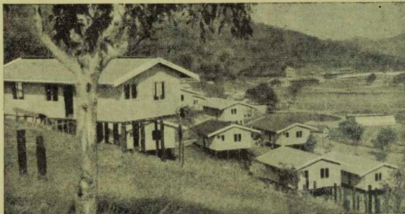
Single men's quarters erected by the Papua-New Guinea Administration at Konedobu, Port Moresby. Painted DAVCO One Coat Metal Paint.
