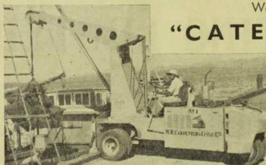
A Hyster Crane at Work on Suva Wharves.
