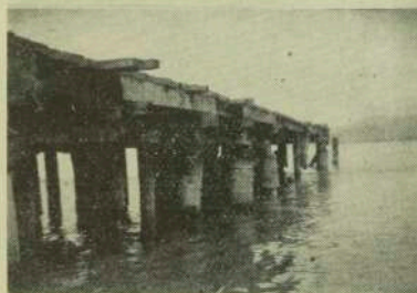
Photographs show: Top left, bridge over Butibum River; top right, another bridge, near Lae. Lower, left and right, wharf at Milford Haven. The round piles in the picture on the left are eaten off at water line and swing with the tide.
