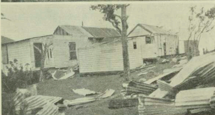
The poignant story of how the hurricane early this year devastated a plantation at Emae, New Hebrides, and destroyed the life's work of the owner was graphically told in the July "P.I.M.": above are photographs showing the extensive damage done on another island, Tongoa, just north-east of Emae. Top.—Only the launch survived when the gale hit the Presbyterian Mission's boat-house. Centre.—Coconut palms, uprooted and flung at random, indicate the cyclone's ferocity. Bottom.—Twisted roofing iron, wrecked walls, and debris littered the yard around this homestead after the hurricane had raced and roared through the plantation.
