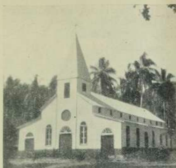
A photograph of the church of the Roman Catholic Mission at Avuvu, Guadalcanal, British Solomon Islands, opened in May, 1938. A peculiarity of the building is that the whole framework is made of native wood, which had to be squared and planed by the natives under the direction of a lay brother, as there was no saw-mill at the station. Dimensions—length, 90 ft.; breadth, 48 ft.; height of the tower, 60 ft. It is one of the biggest timber churches in the Solomon Islands.
