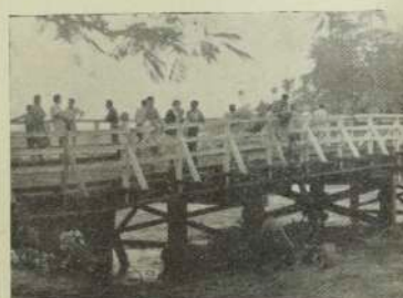
Scenes near Apia after the heavy rains in Western Samoa in January and early February. Floods were general and the damage very extensive.
