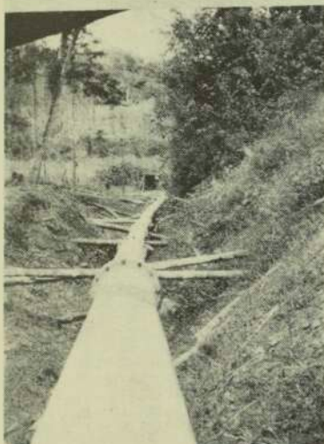
Here are shown photographs of the new workings of the Sandy Creek Gold Shuiling Co., near the mouth of Sandy Creek and the Bulolo River, New Guinea. The pictures show pipe line, nozzle heads and elevator. At night, the workings are flood-lit by electric light.
