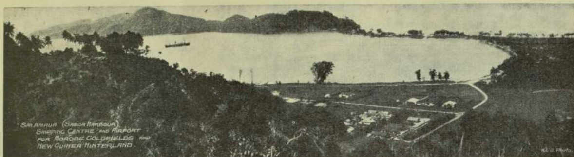
Salamaua harbour and isthmus, seen from the mainland. The present town is on the isthmus, and the aerodrome is away to the right. In the foreground are new buildings on Kila Point. The foreshore on the right is part of the large swamp, which it is proposed to drain, in order to lay out the new town.
