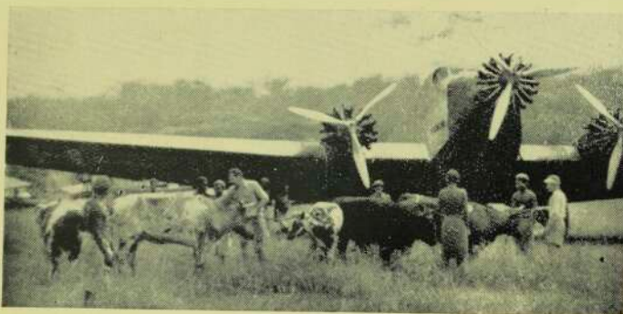
The above photograph shows how aerial transport is assisting in the establishment of a pastoral industry on the Morobe tableland in New Guinea. These dairy cows have just been unloaded from one of Guinea Airways' freight-carrying aeroplanes after being transported from the coast for a dairy farmer near Wau.
