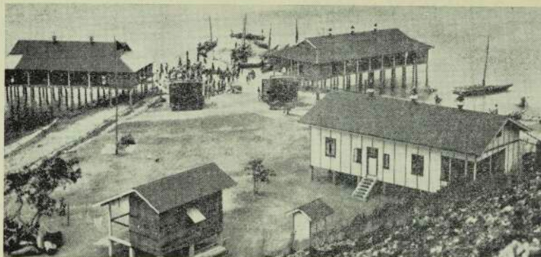
The new hospital buildings at Gemo Island, constructed over the water's edge, which were officially opened in October. In the right foreground is the fibro-cement dwelling of the sister-in-charge.
