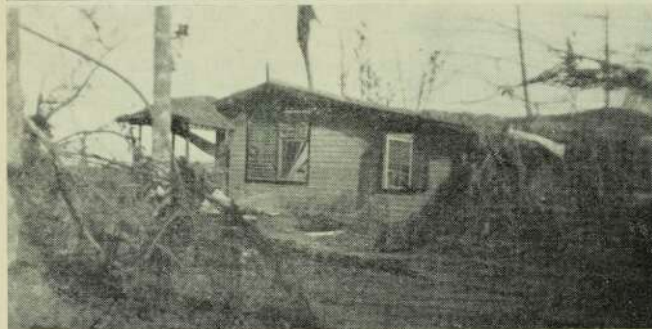
Mr. Syd. Costelloe's house, Kokopo Road, after much excavating had been done.
