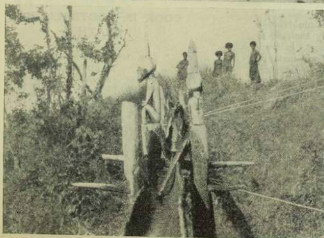
Lower: The old water-race, of hollowed logs, which carries the water across the gully. Note the carved figures which guard the structure.
