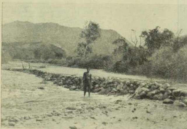
Top: The dam, on Uruam Creek, made of stones, and the interstices kept filled with mud and grass.
