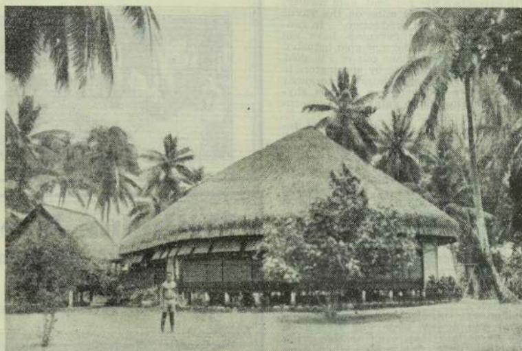
The residence of the late F. W. Murnau, in Tahiti, which was destroyed by fire on August 25. Photo.: Paul Nordmann.
