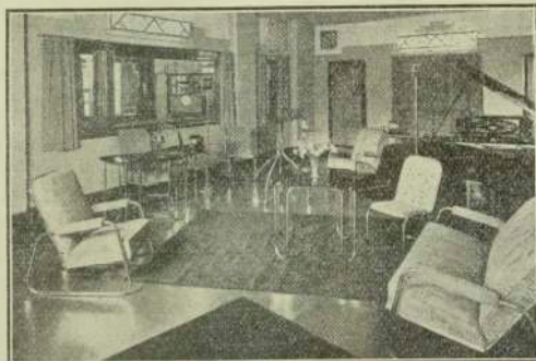
Radio Station 2UW, Newlands Steel Furniture
