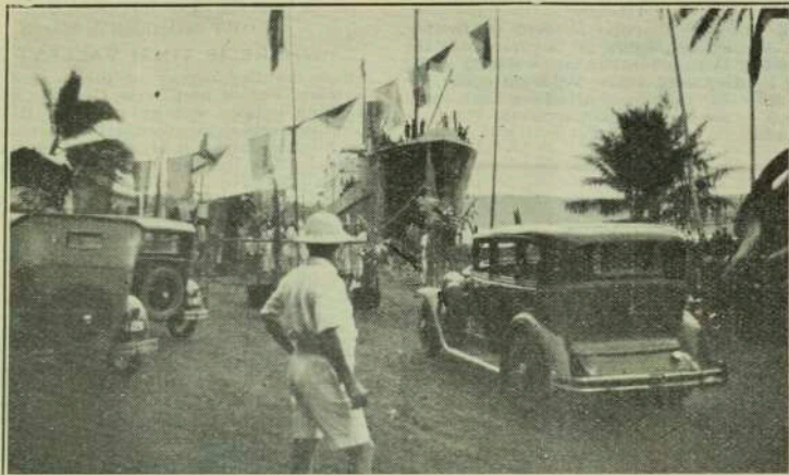
Photograph taken on January 18 last, when the new slipway built near Rabaul, New Guinea, by Messrs. W. R. Carpenter and Co. Ltd., was officially opened by the
