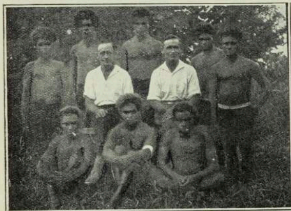
The builders of the Hospital, Messrs. A. and H. Kohnke, of Brisbane, and their team of native carpenters.
