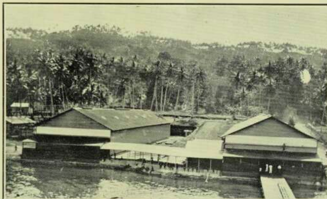
The large copra stores, complete with modern equipment, erected on the waterfront at Rabaul by W. R. Carpenter and Co., Ltd.
