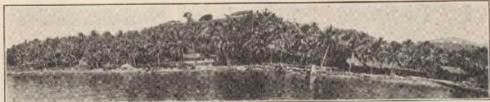
The landing station at Suva, Melauia, F.S.I., which felt the full force of the earthquake. The Matson Company's buildings (shown above) and wharf (on right hand corner) were severely damaged.
