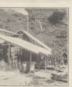
A photo of the Day Dawn (New Guinea) Ltd. plant, taken shortly before crushing commenced. The mill itself can be seen on the left. The entire machine is about 10 ft. away. All this machinery was transported from the coast by aeroplane.
