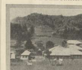
The Cable Station at Norfolk Island, situated at Anna Bay, seven miles from Kingston. It was established in 1922.
